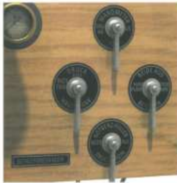
The fuel switches unit.
